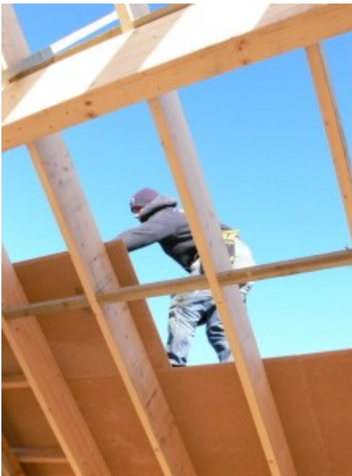
PAVAROOF Installation at Trevone Bay, Cornwall
