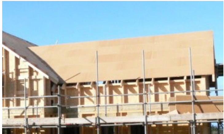
PAVAROOF Installation at Trevone Bay, Cornwall
